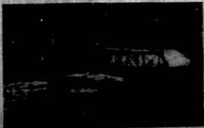
Native bridge on the Chania River.
