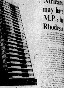
A view of the 22-story hotel of Harp in London, showing the section which collapsed after an explosion. Three people were killed in the incident which happened early in the morning. A hundred of the residents were still in bed.
