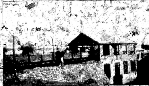
Sorting shed, upper level.
