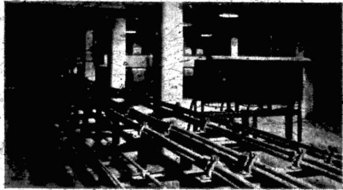
Electricity Authority of Cyprus. Cable basement in Dhiekelia Power Station.
