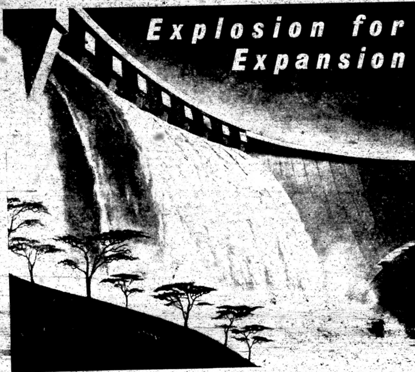
BEFORE THE BLAST —the coffer dam before it was breached, loaded with 4 tons of explosives in 40 holes.
