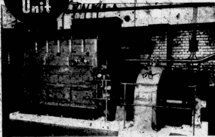
The photograph shows a Petter Super-charge Engine installed in a factory.
