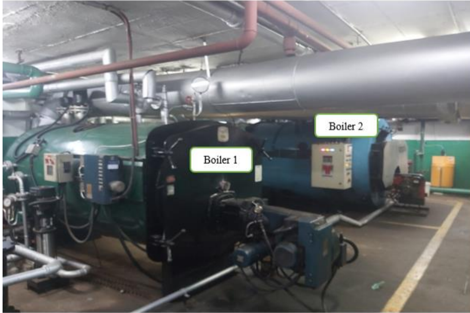
Figure 4. 2 Existing Hot Water System
