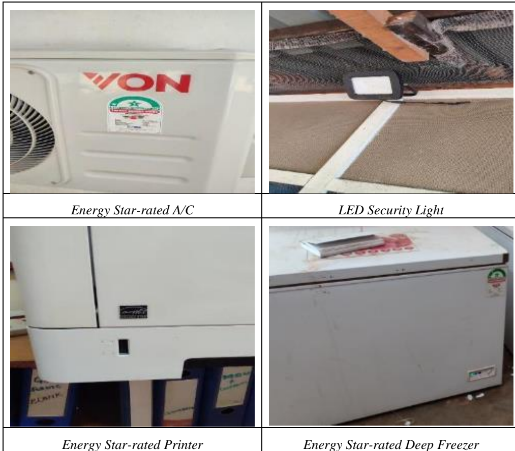
Figure 6.3: Implemented Energy Conservation Measures
