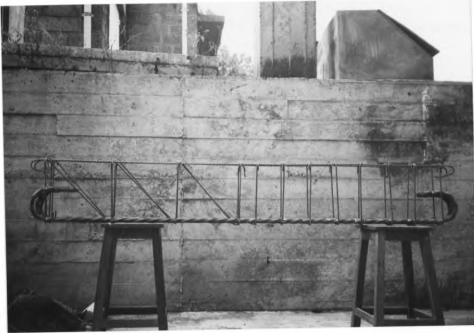
(a) Arrangement of reinforcement
