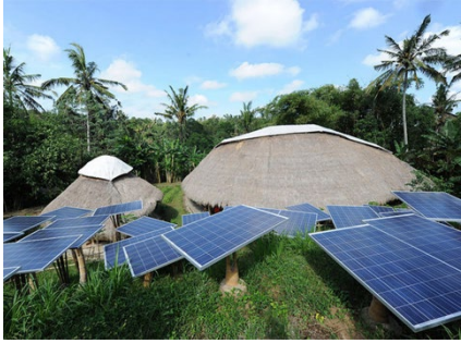
Figure 33 Photo Voltaic cells in Green School Bali Source: Green school Bali.
