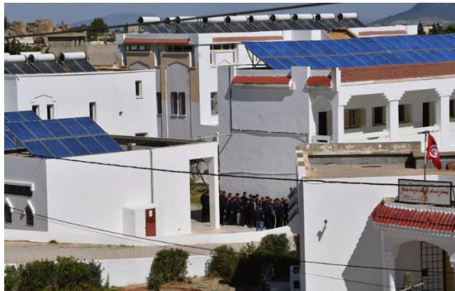
Figure 36 Solar panels installed on the roofs of the school. Source: FETHI BELAID AFP
