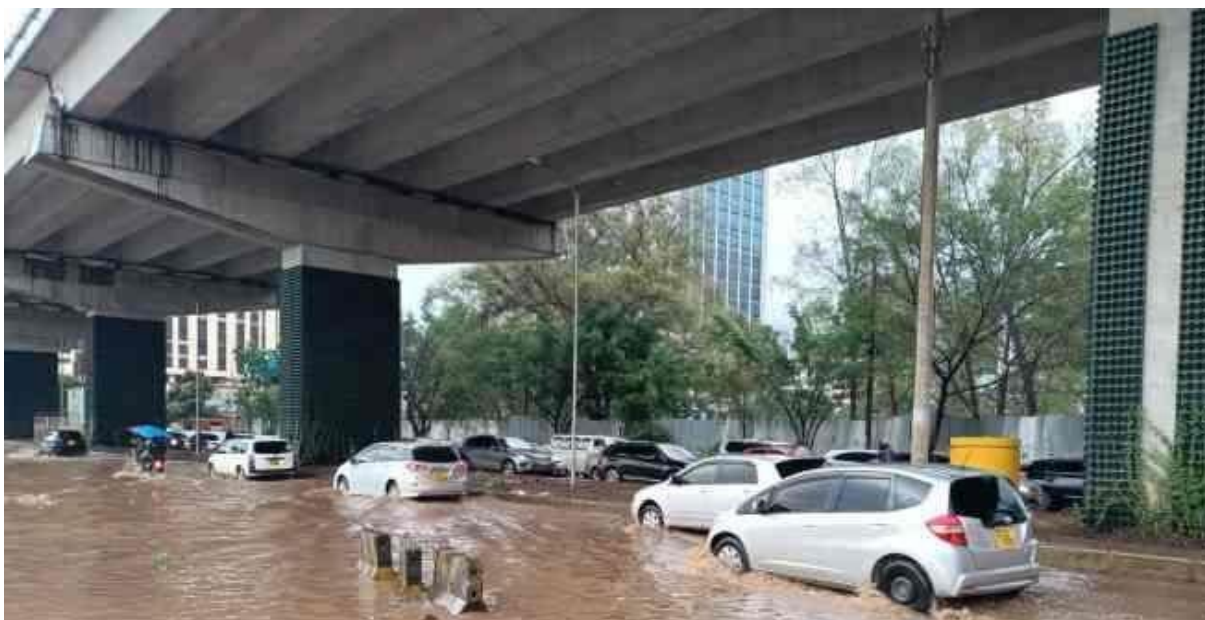
Plate 8: Flooding along Uhuru Highway
