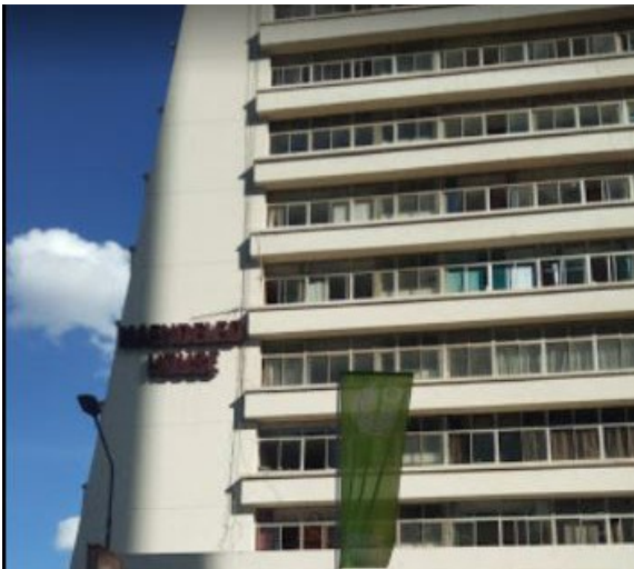
Fig2.6. Horizontal shading on Maendeleo House, Nairobi Source: Google Earth.
