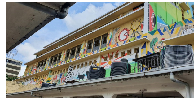
Fig2.10. Horizontal sun shading devices at City Market, Nairobi. Type A according to fig 2.8. Source: Author
