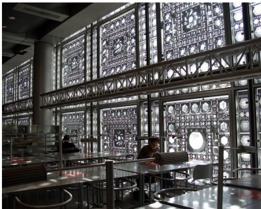
Fig 5.8. Representation of the mushrabiya screen in the robotic shading screen of Institut du Monde Arabe.
