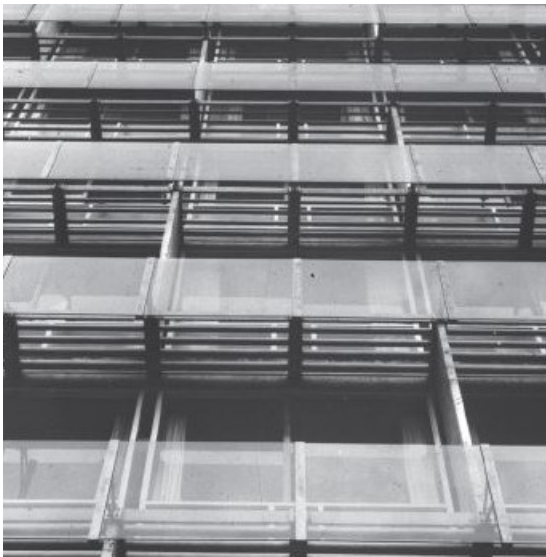
Fig2.1. Sun shading device on the exterior of Unesco House.
