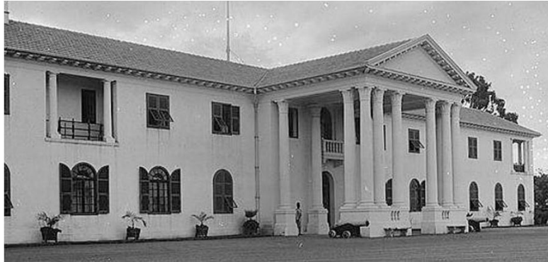
Fig 4.22. State House in 1934 designed by Sir Herbert Baker.
