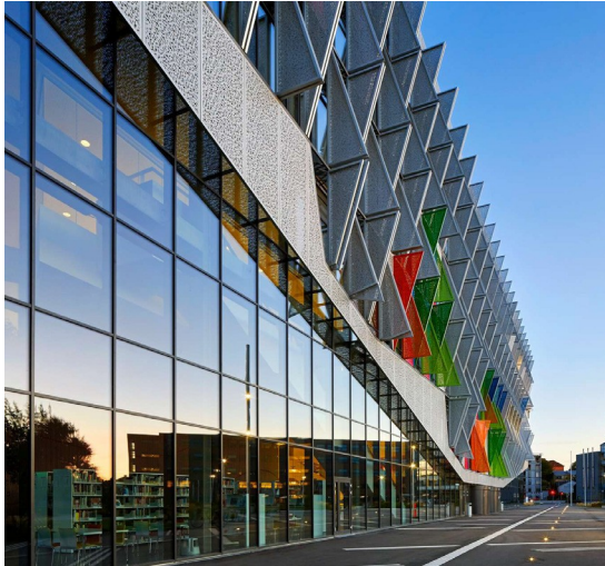
Fig 5.7. Creative Climate responsive facade of SDU- Kolding University of Southern Denmark.
