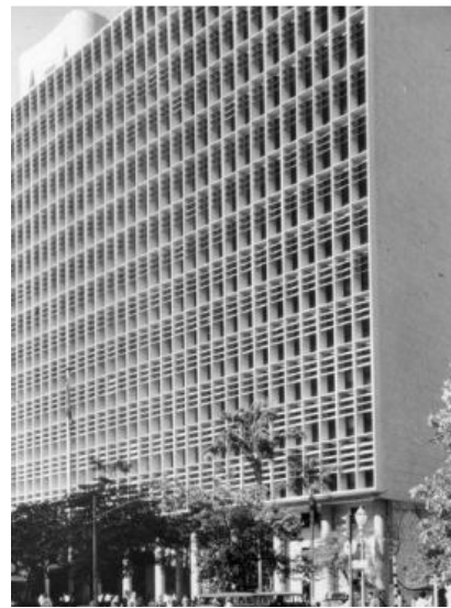
Fig 2.35. Sun shading devices on the Ministry of Public Health Building in Rio. Source: www.foundationlecorbusier.com
