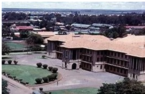
Fig4.28 Aerial view of Railways Headquarters
