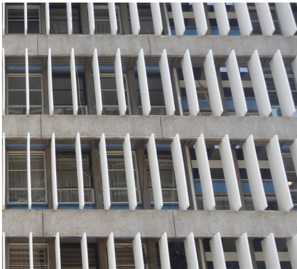
Fig2.11. Vertical shading on Jogoo House B Source: Google Earth.
