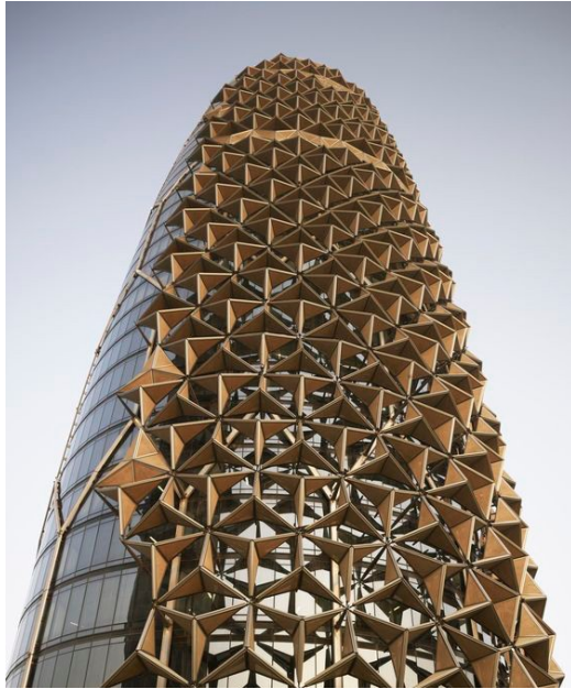
Fig5.6. Al Bahar Towers, Abu Dhabi with automatic shading facade that opens and closes in response to the sun's movements.
