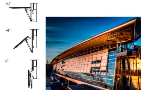
Fig2.16. Perforated metal rotating shading system at Zurich airport. Source: Dakheel et al. (2017)
