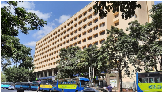
Fig5.4. Recessed windows of Kencom building facade act as secondary sun shading feature.
