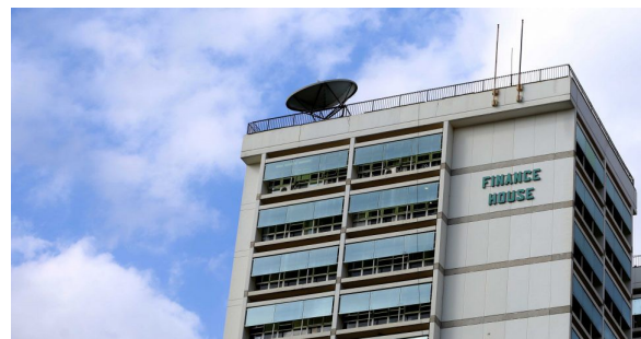
Fig2.9. Horizontal sun shading devices at Finance House, Nairobi. Type J according to fig. 2.7 Source: Flickr.com
