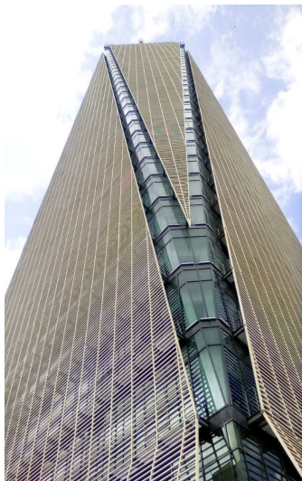
Fig 4.43. Britam Tower veil sunshading device.
