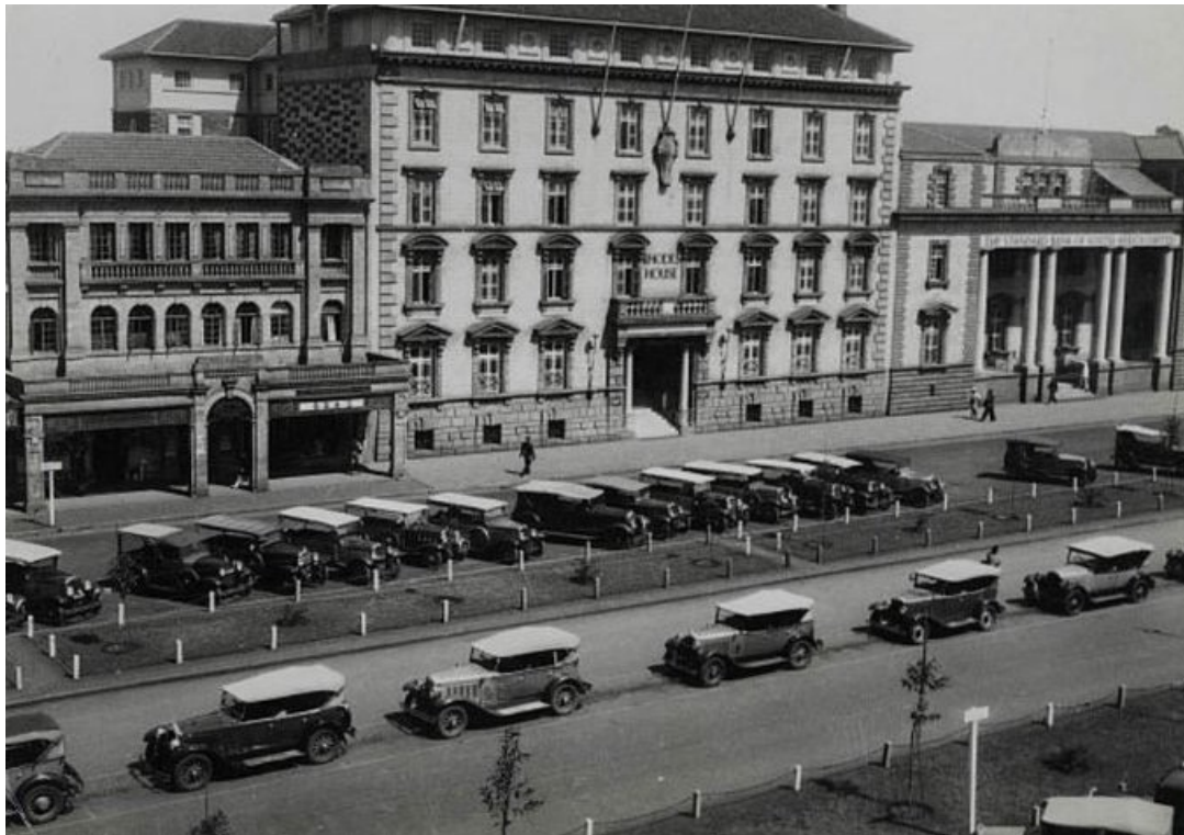
Fig4.26 Delamere Avenue showing Stanchart, Panafic House and Westminster House from right to left. These three buildings still stand today as a reflection of the construction in the 1930s.
