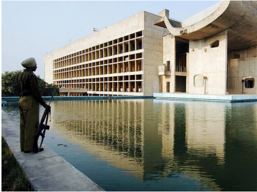
Fig2.34. Brise soleil in Chandigarh designed by LeCorbusier. Source:the guardian
