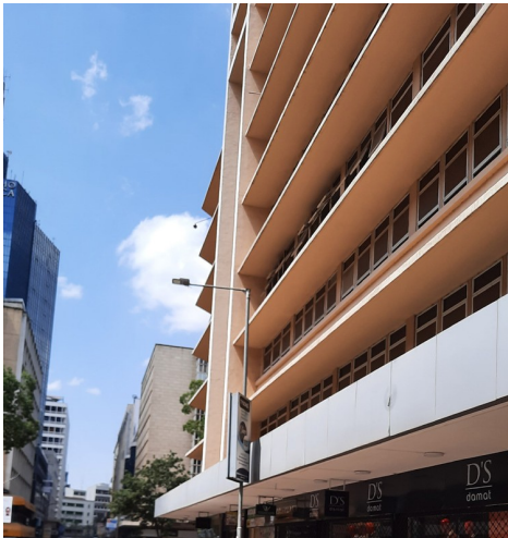
Fig5.2. Horizontal shading devices on Jubilee house.
