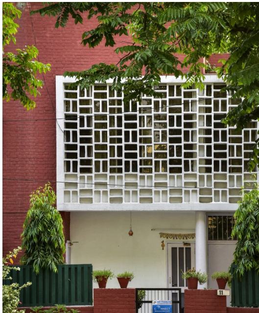
Fig 2.37. Building in Chandigarh's sector 22 designed by Maxwell Fry and Jane Drew showing interpretation of jaalis .
