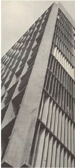
Fig2.45. Building showing different sun shading devices for different orientations. Source: Olgyay & Olgyay (1957)
