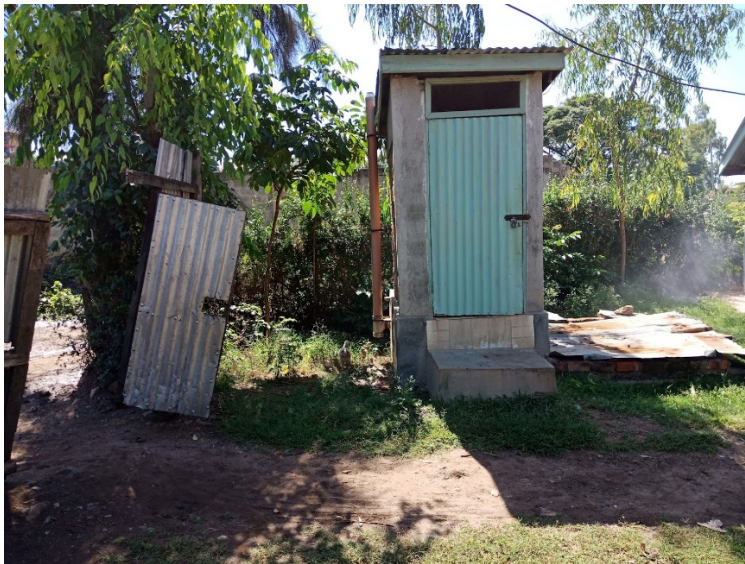
Figure 4: A hand dug well situated adjacent to a pit latrine. The water is under great threat of contamination.
