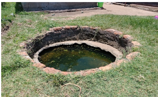
Figure 3: An unprotected hand dug well.
