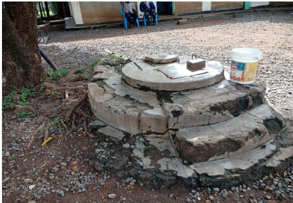
Figure 2: A protected hand dug well with intact well head and well cover.
