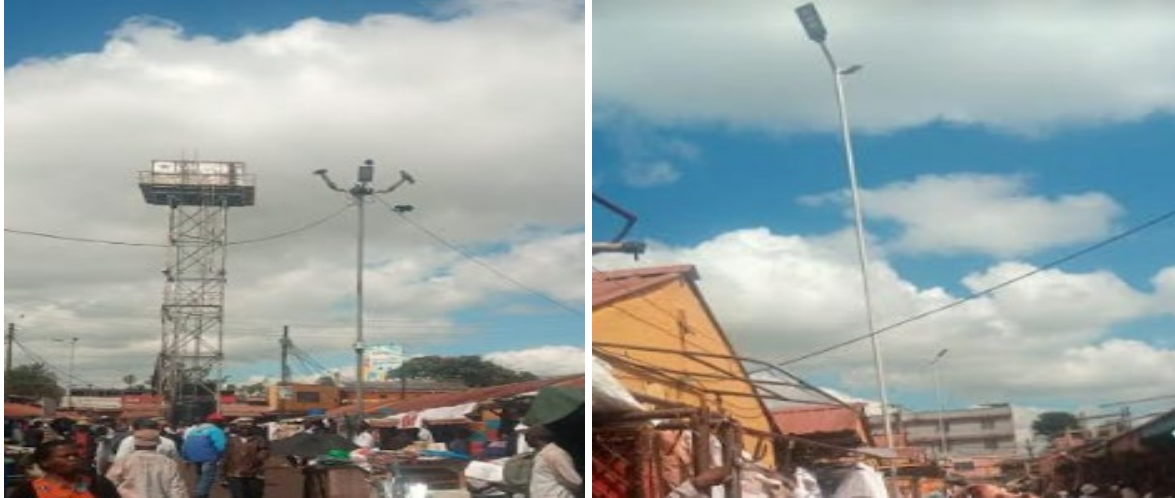
Picture 15 State of Street lighting in Burma Market, Source: (Camera photo 2024)
