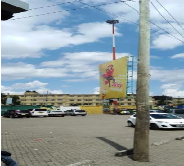
Picture 8 High mast lighting in Kariokor Market, Source: (Camera photo 2024)
