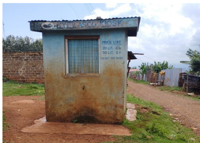
Figure 5-1: Transformer Water Supply Point
