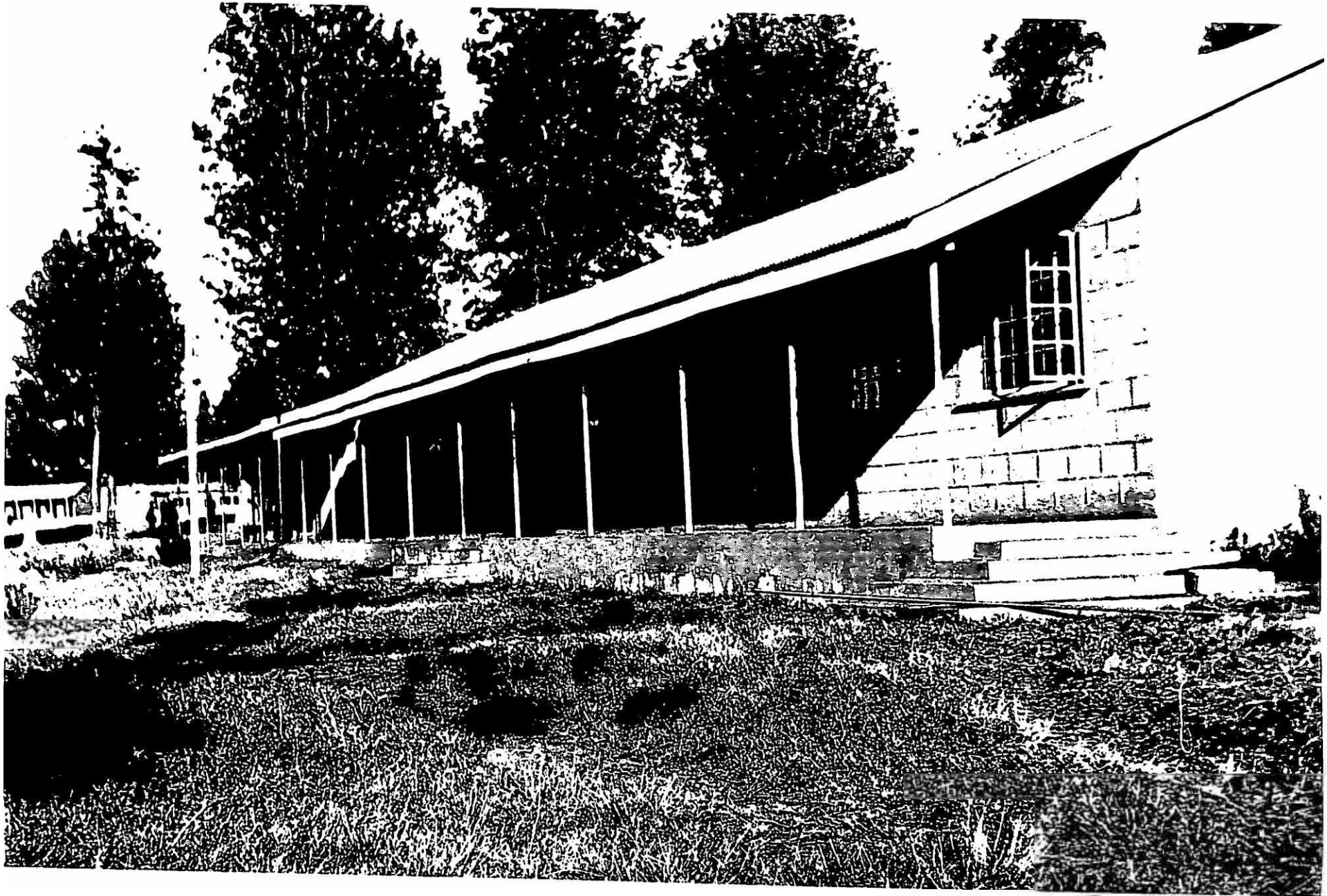
TYPICAL URBAN PRIMARY SCHOOL - ELDORET MUNICIPAL COUNCIL
