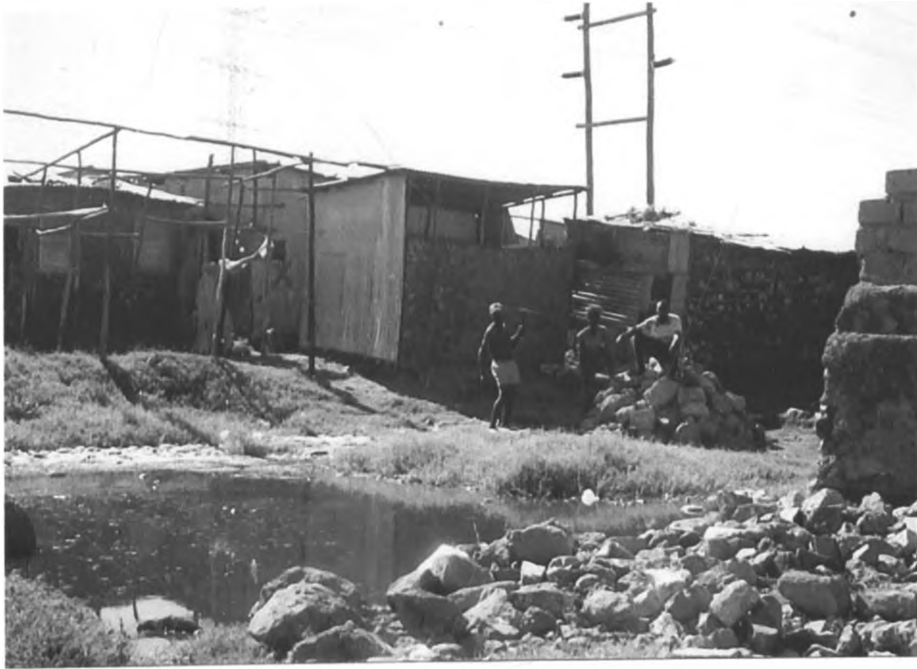
Fig. 4.8 Stagnant Pool of Water next to Housing Structures in Mukuru Kwa Njenga
