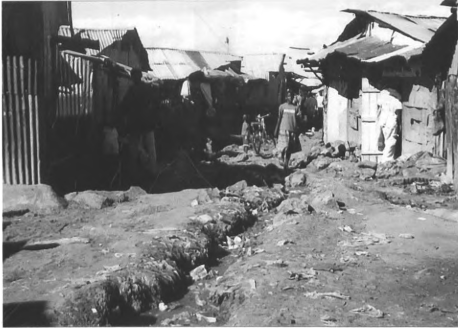
Fig. 4.9 Water Gullies on a Road in Mukuru Kwa Njenga
