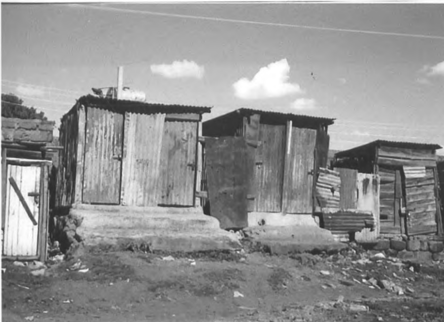
Fig. 4.2 Pit Latrines in Mukuru Kwa Njenga (see the poor state of repair)
