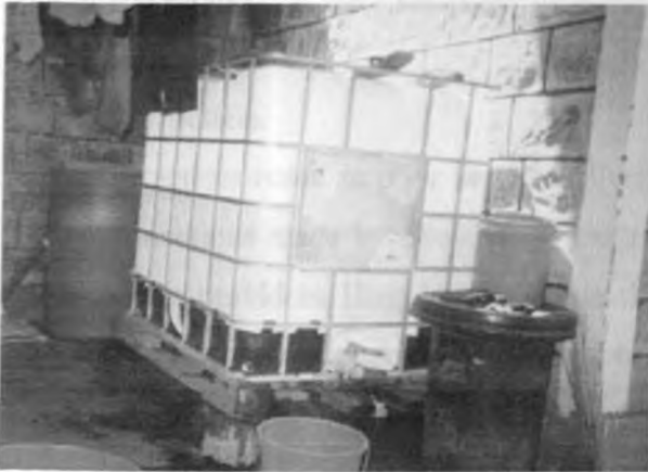
Photo IX. Water storage tank in a house compound Umoja II
