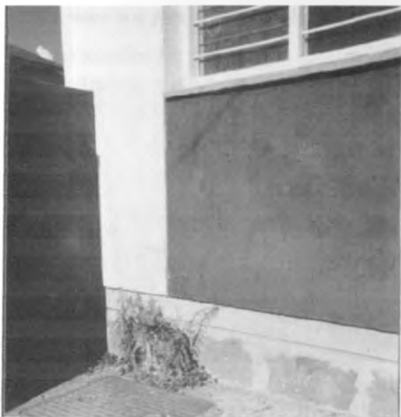
Photo VI. Position of water meter within a compound in Prudential estate
