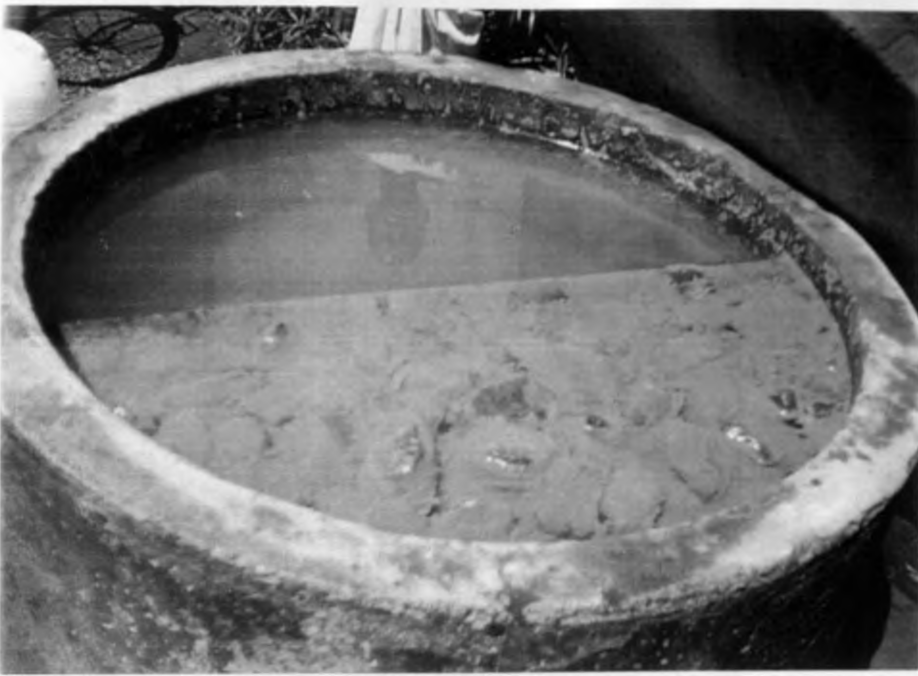
PLATE 5 Siging Plant two days after backwashing
