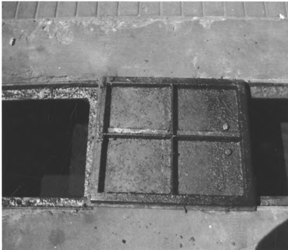
Fig. 11: This shows proper used oil handling.
