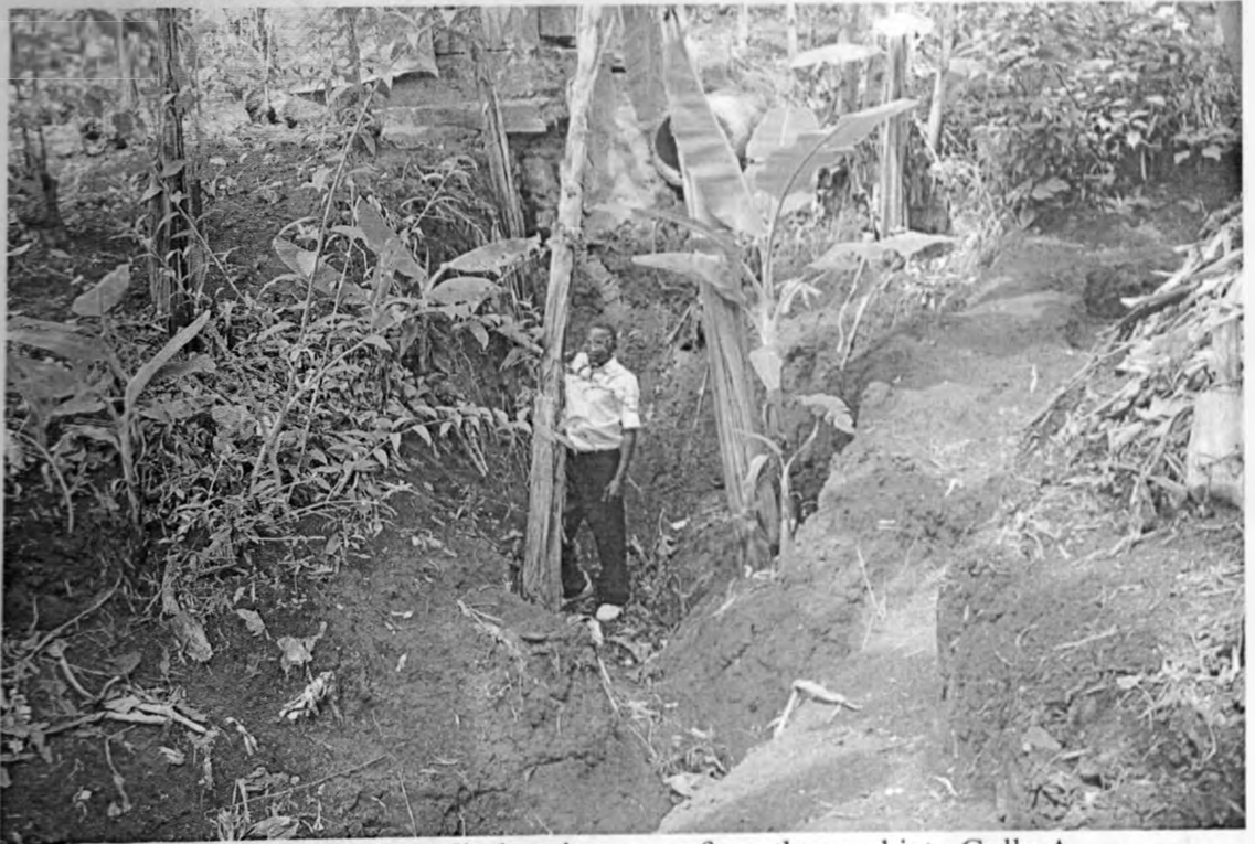
Plate A6: Culvert discharging water from the road into Gully A
