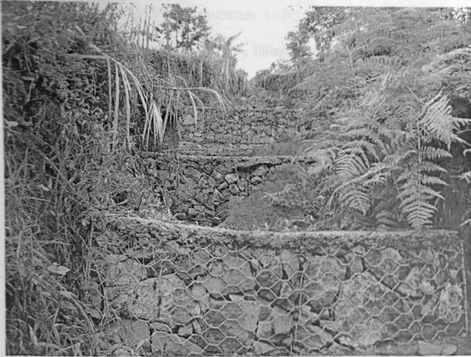
Plate 4.5: Gabions put in Gully B to control erosion
