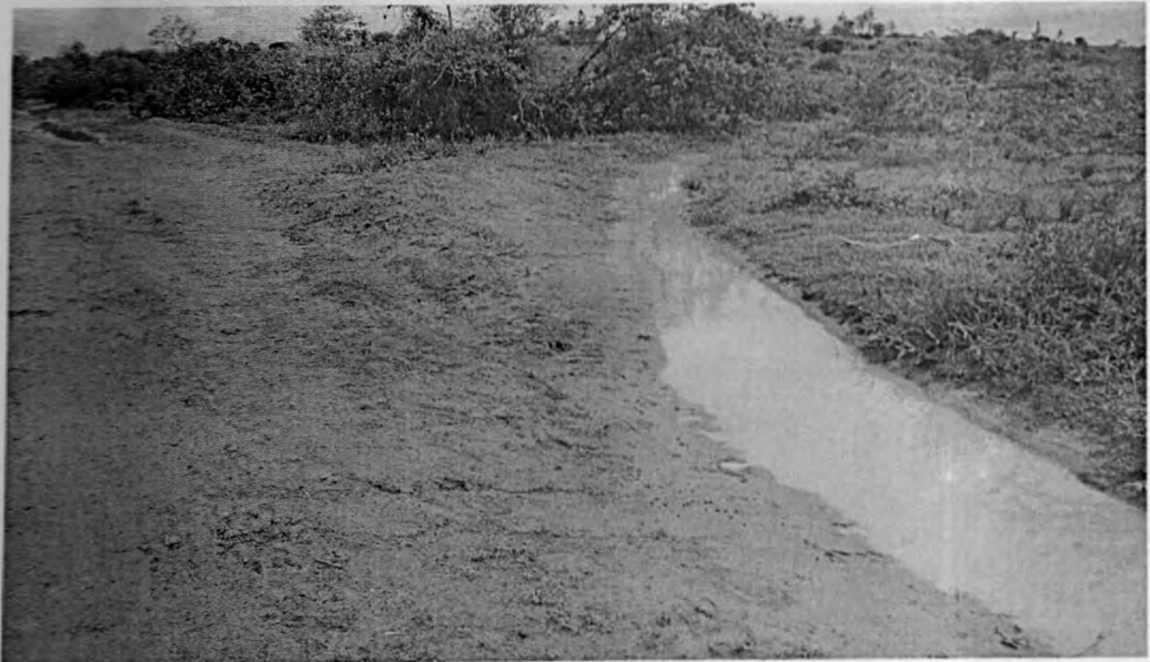
Plate A2: Water directed into the farms through mitre drains
