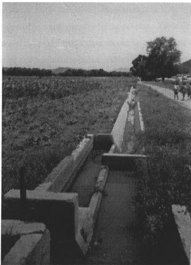
Plate 1 Weedy and silted check divider in block A: Nyanyadzi scheme
