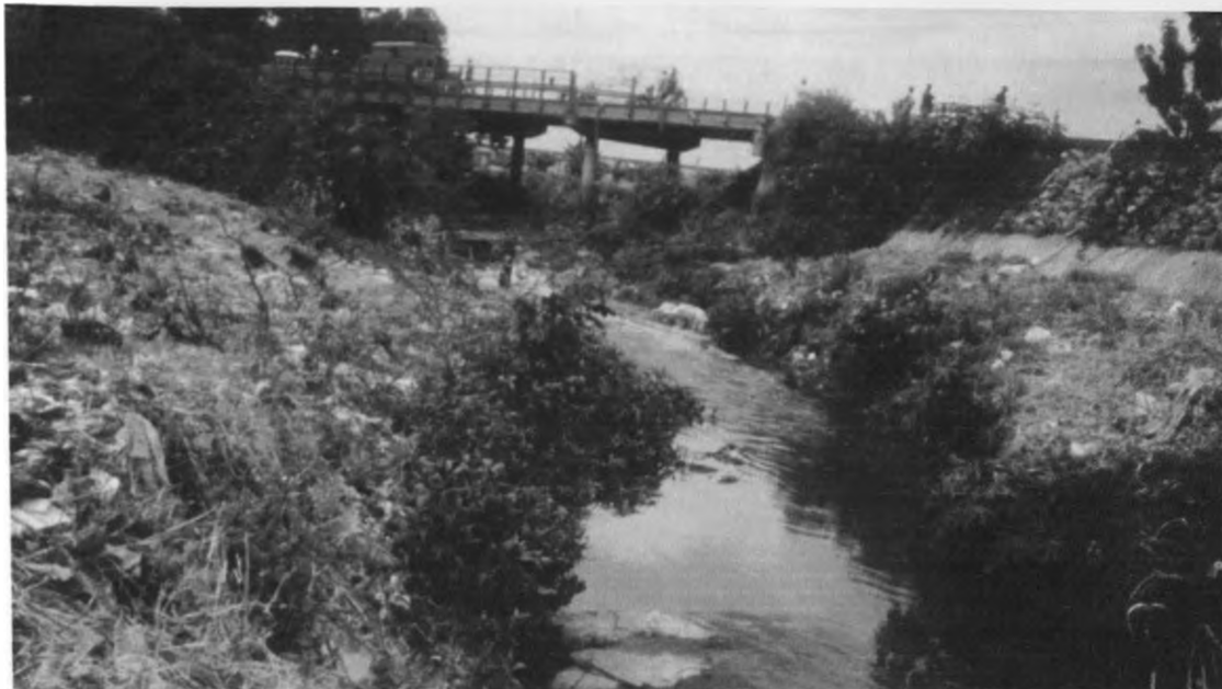
Plate 1: Globe Cinema round about before heavy storm (dry season)- notice heaps of garbage and solid wastes on the river channel and banks.
