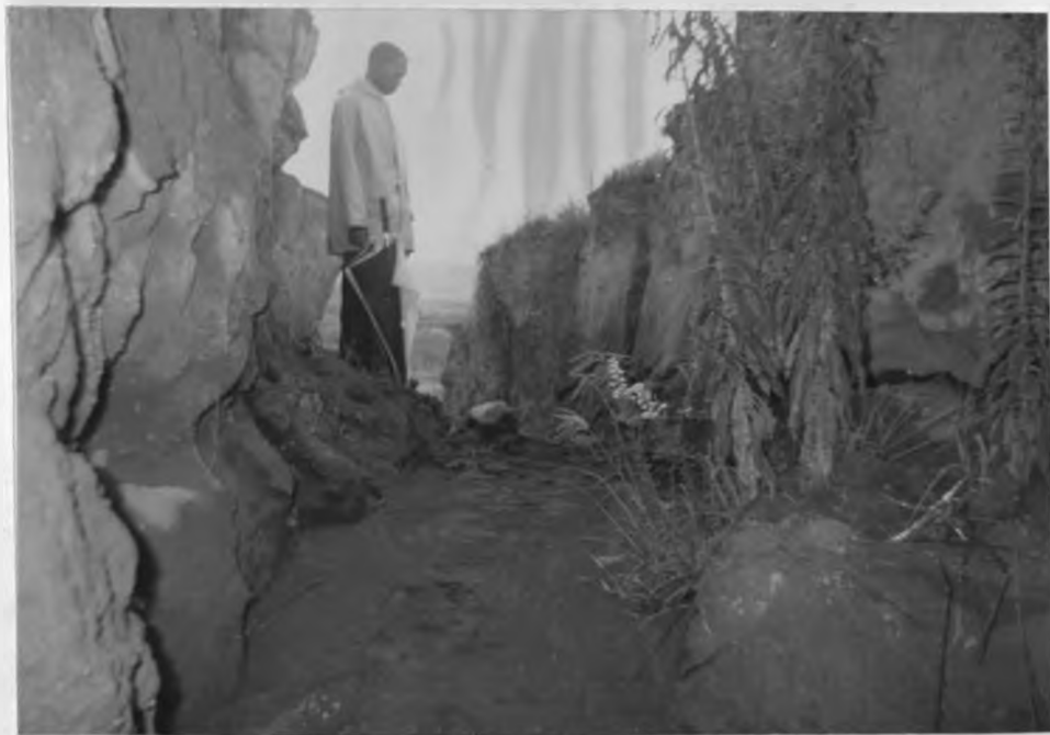
Plate 10. Deposition upstream of loose stone check dam no. 2 at the end of the first rainy season.
