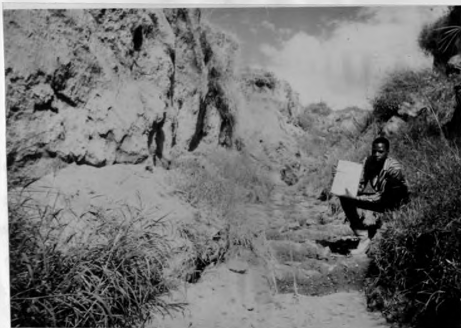
Plate 9. Scoured bed of the grassed parabolic waterway of gully A after the first rainy season.
