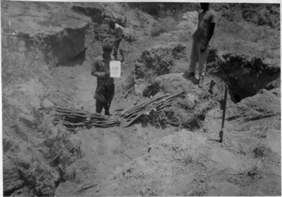
Plate 12. Brushwood check dam no. 2 after the first rainy season. Notice key failure on the right.
