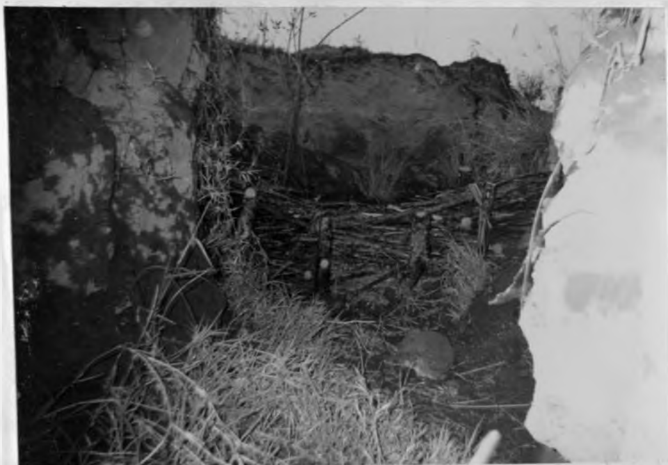
Plate 11. Brushwood check dam no. 1 shortly after the first runoff event during the study.
