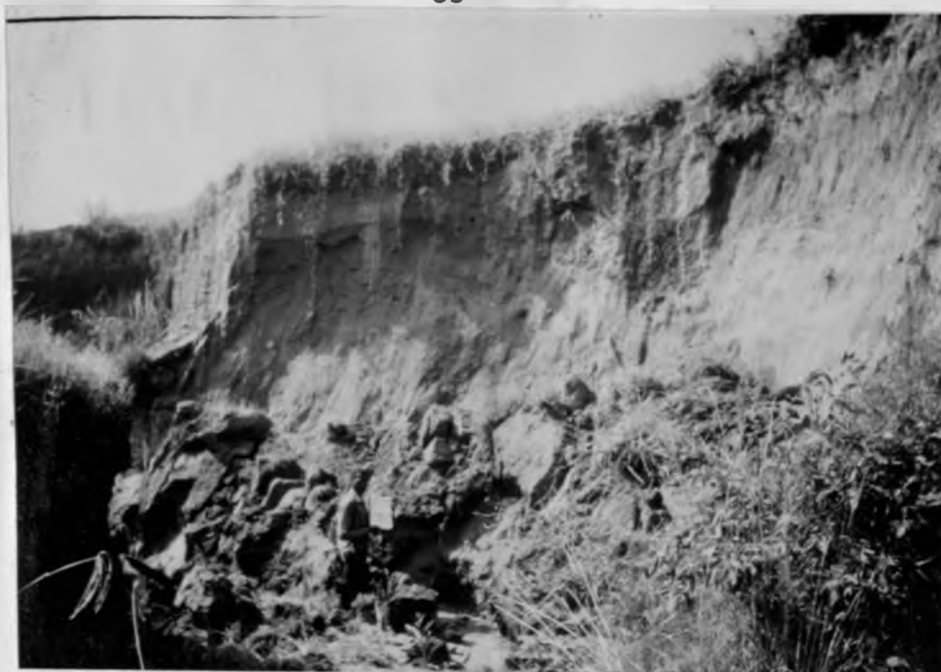
Plate 4. A major sidewall collapse at a deep section (19-20) of gully A.
