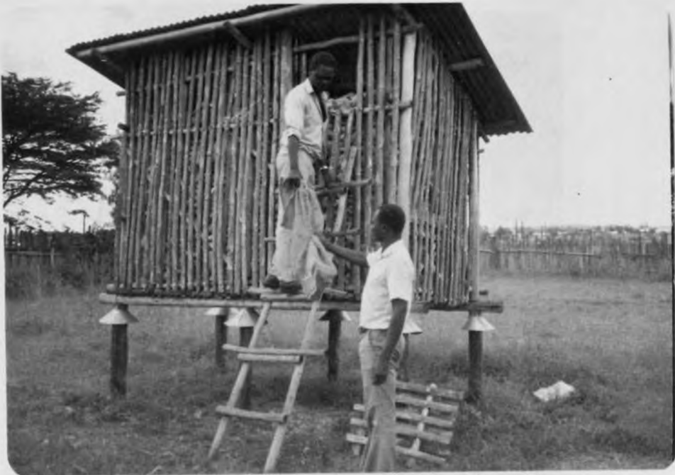
Figure 5: Ventilated maize crib
