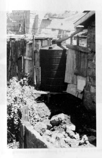
Figure 8: A photograph showing an improperly erected plastic water tank in Kikuyu.
