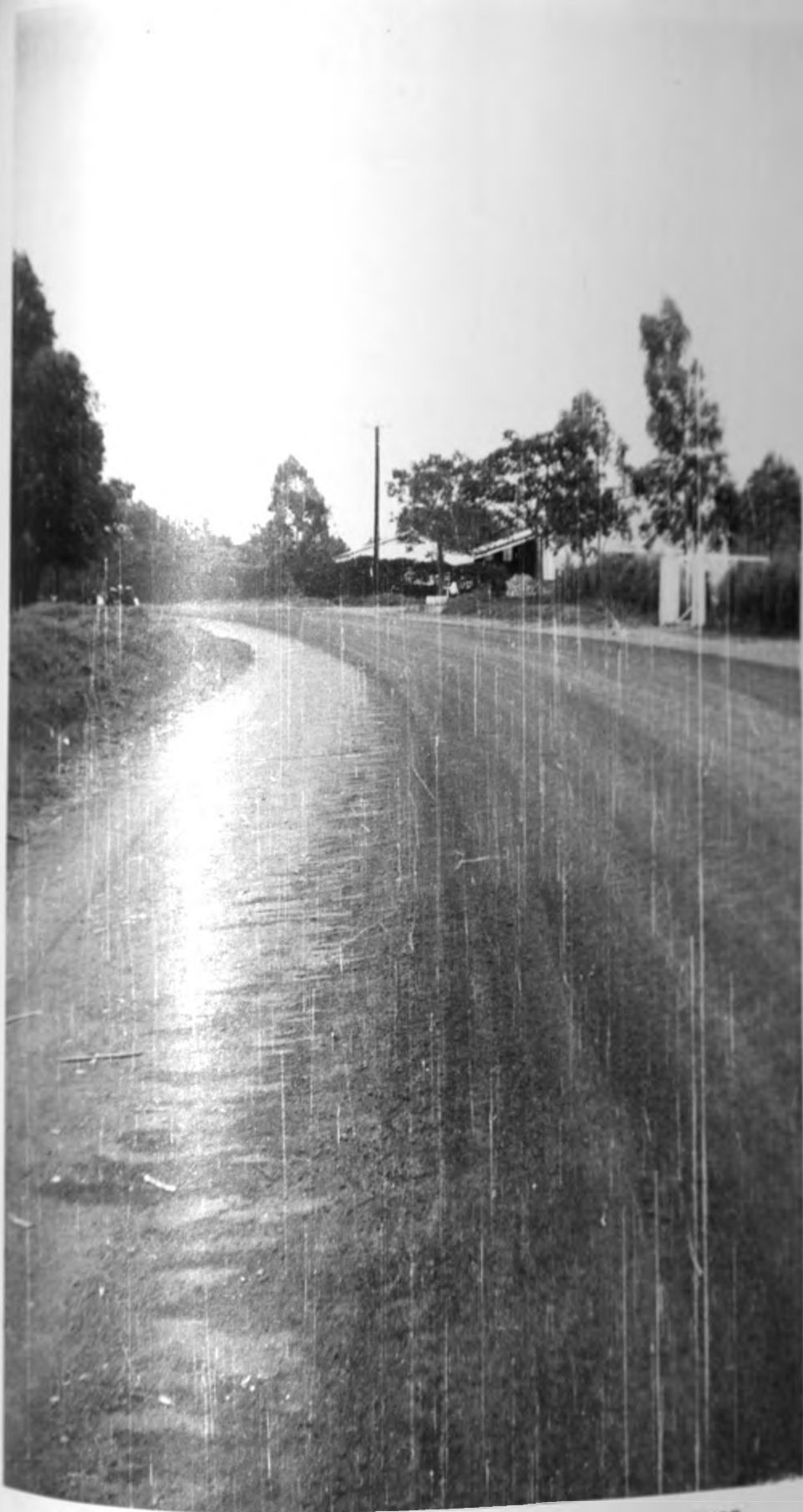
Plate 17. A road in the Mumias factory residential area covered with molasses in order to reduce the dust.
