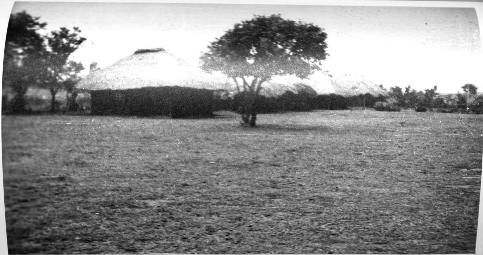
Plate 8. A primary school in Mumias sugar belt constructed by the sugarcane outgrower farmers through harambee spirit
