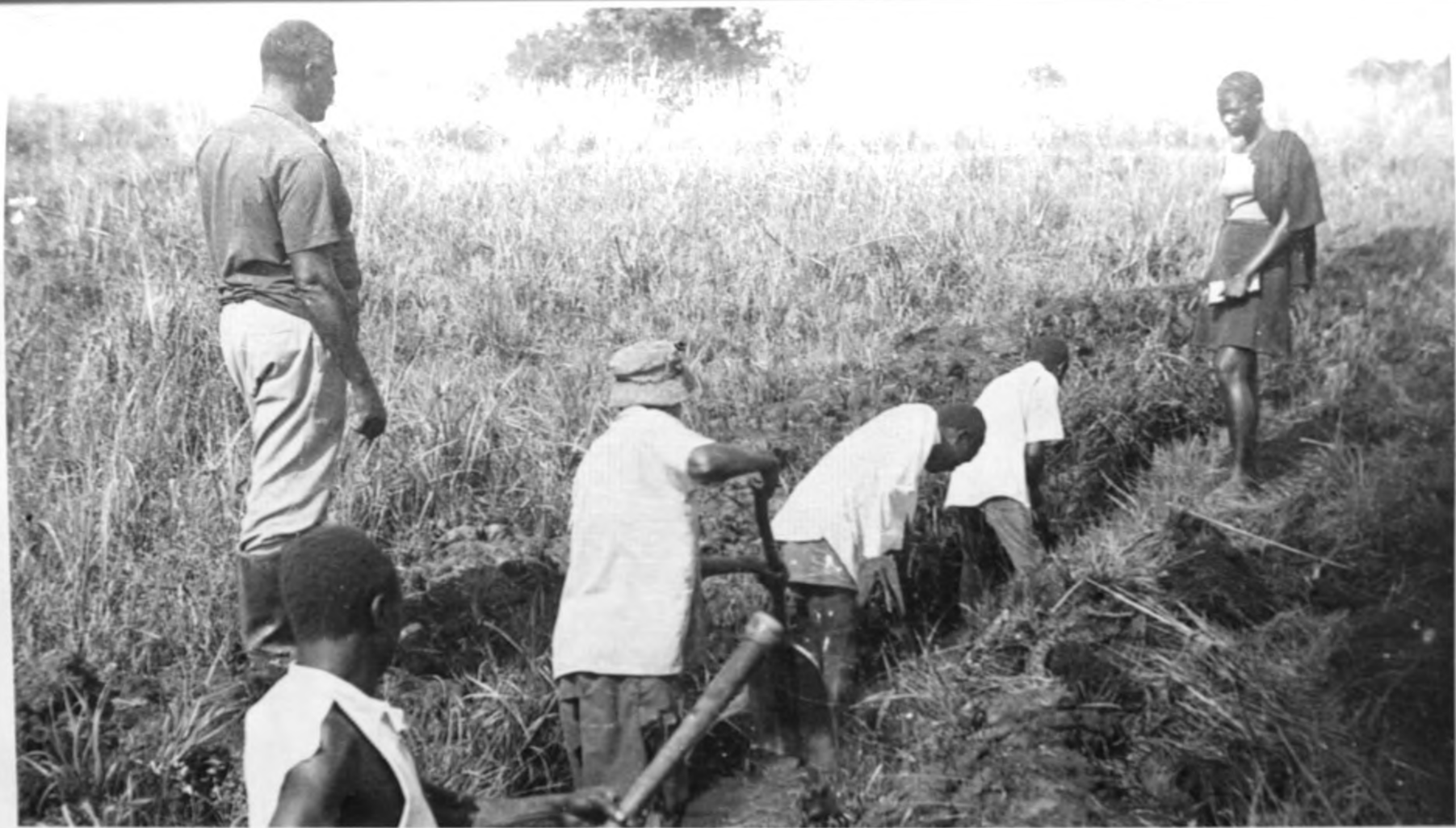
Plate 1. A piece of land being drained for sugarcane plantation.
