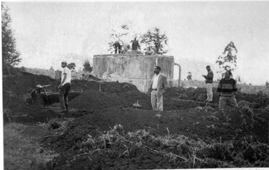
Plate 5.6: A picture showing the old water tank and the preparation of the site for the new water tank in Gitangu ISS, Kiambu District, Kenya, June 2000.
