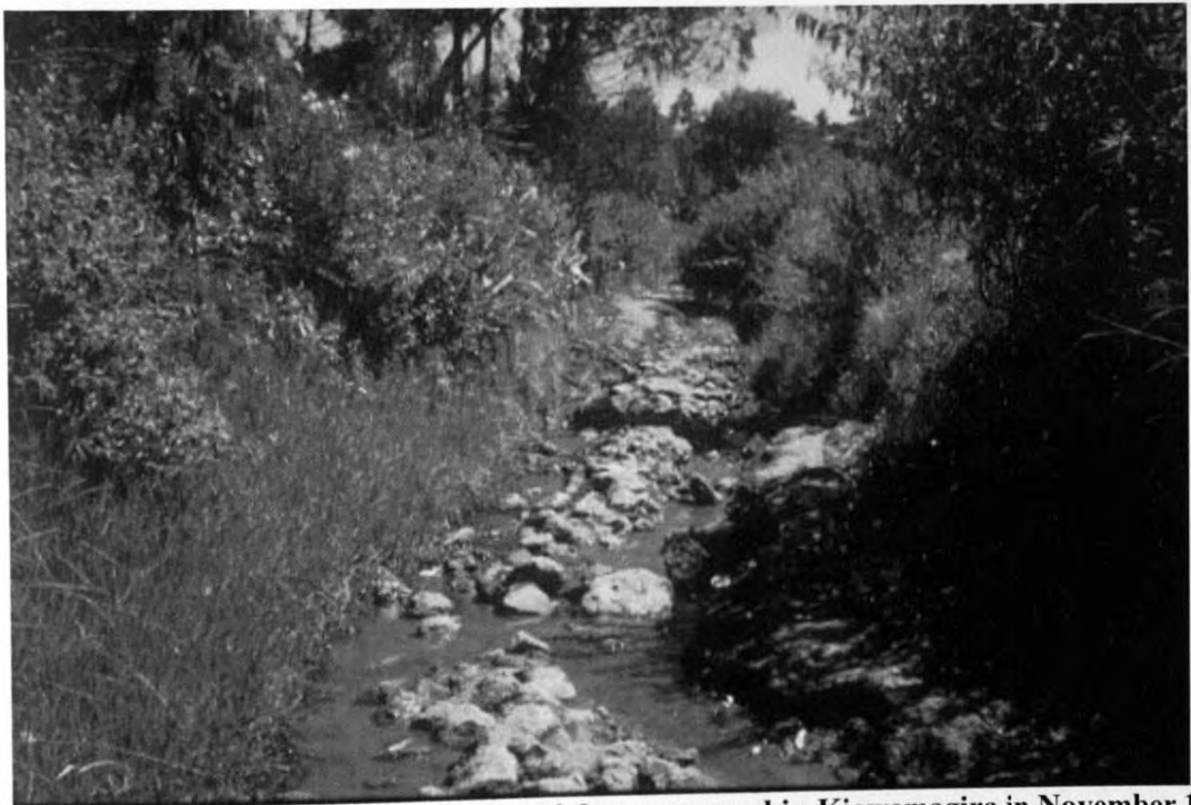
Plate 5.4: A picture showing the condition of the access road in Kiawamagira in November 1997 after the initial attempts by the community to repair it.
