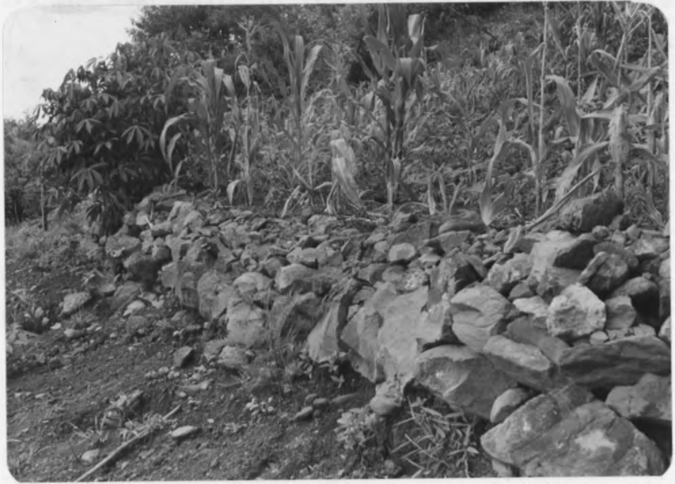
Plate 13. Removal of stones for bunding may accelerate erosion at the lower edges of bunds.
