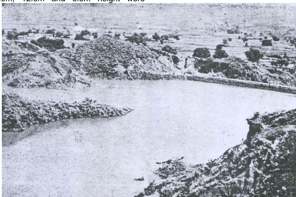
Figure 2: Site showing catchment, an earthen dam, reservoir and command area.
