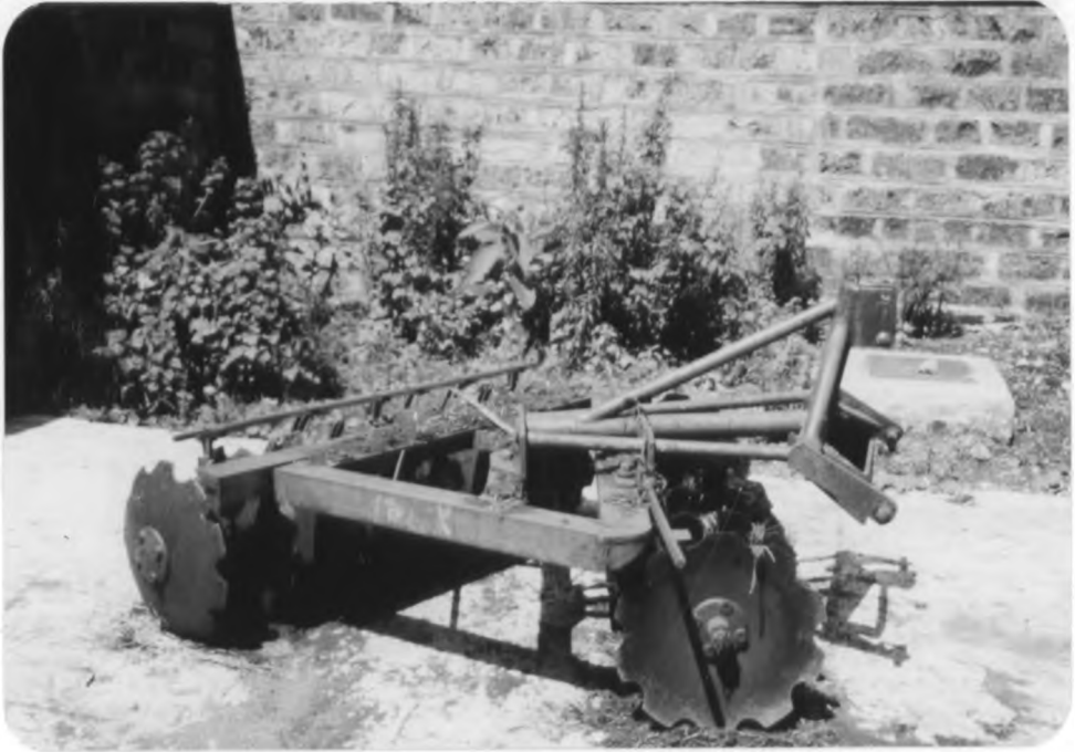
Plate 9 The offset disk harrow used for conventional tillage treatments
