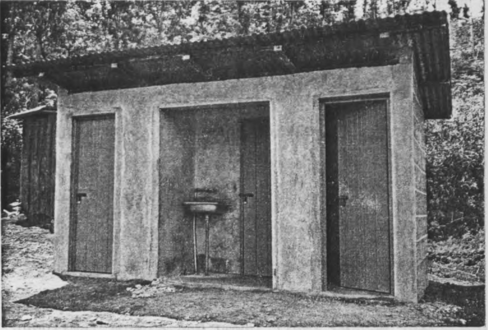
(a) A modern sanitary facility.
