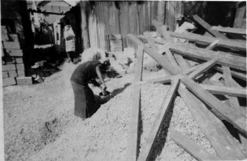
Plate 3.3q: Aggregate batching.
