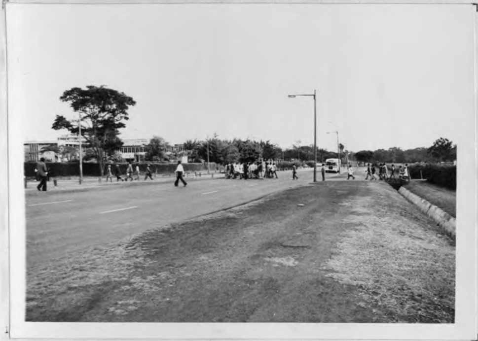
PLATE-10 Uncontrolled pedestrian crossing
