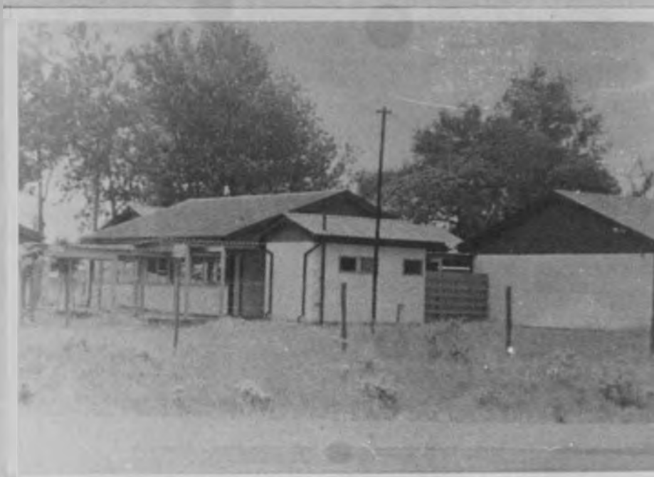
DANDORA PROJECT OFFICES
