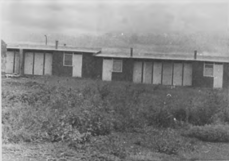
WET CORE AND ONE ROOM PROVIDED
