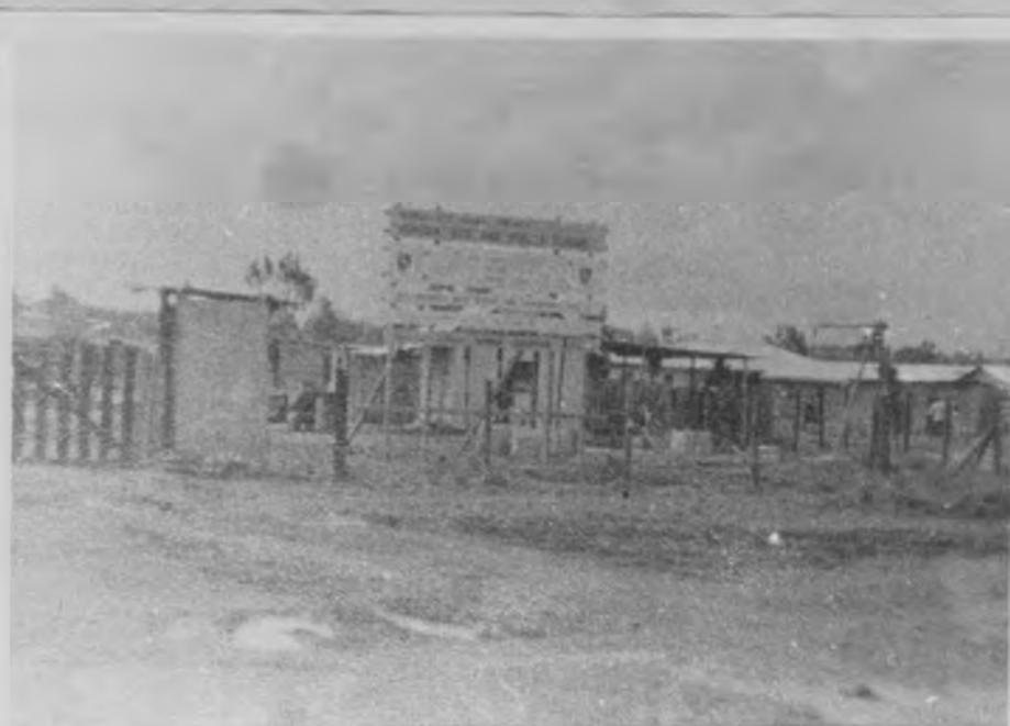
MATERIAL SHADE AT HURUMA
