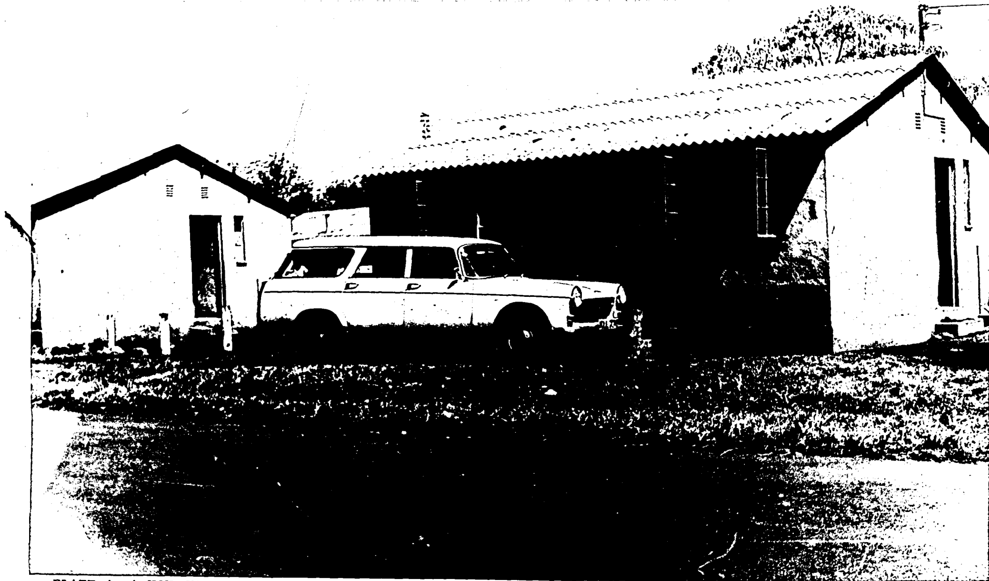
PLATE 4 A HOUSING UNIT IN ONDIEK ESTATE OCCUPIED BY A MIDDLE INCOME EARNER. The occupants are in the house but the main door is left open apparently to keep watch on the car parked in front of the house. The house number on top of the door, R2/205 was invaluable for sampling purposes.
