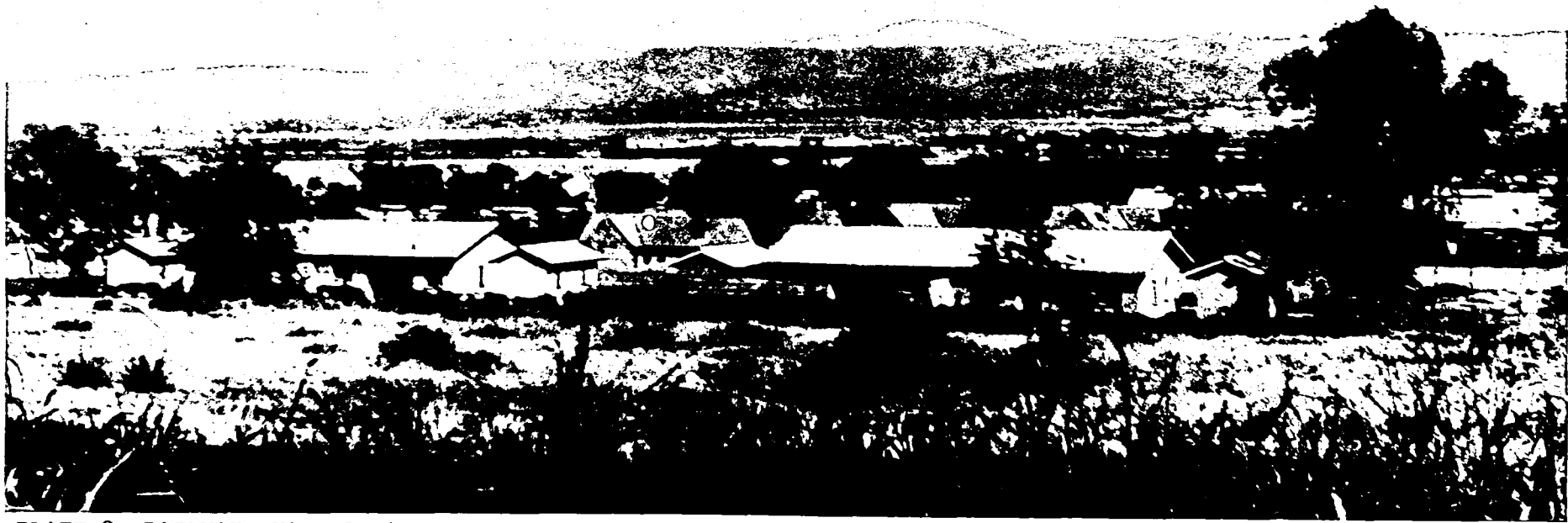
PLATE 8 RAILWAY QUARTERS ADJACENT TO MLIMANI AREA IN KISUMU. These are occupied exclusively by the East African Railways Corporation employees. In the immediate background is the lake and the new industrial area. On the far background can be seen the Kisian range and Maseno and Bunyore hills.
