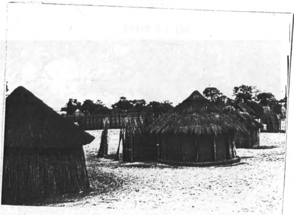
USE OF LOCAL MATERIALS FOR HOUSING IN MAUN - POLES, REEDS, MUD, GRASS
