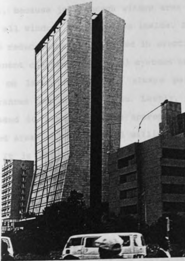
Plate 6.2. Photograph of Cooperative Building. Building with permanent gantry for cleaning purposes.
