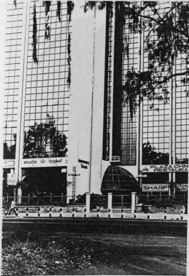
Plate 6.1. Photograph of Anniversary Towers. Building with permanent gantry for cleaning purposes.
