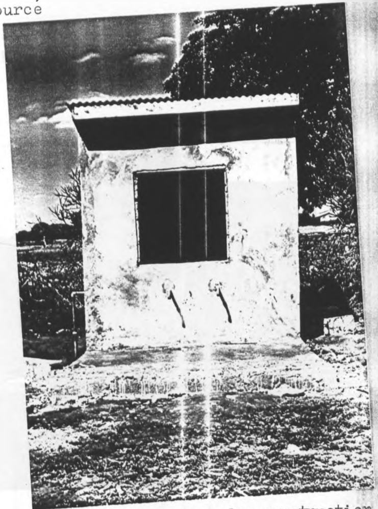
New water facility under construction Kithimani
