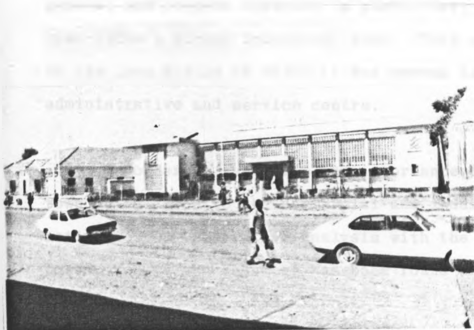
Plate 7: Part of the Banking facilities in the town.
