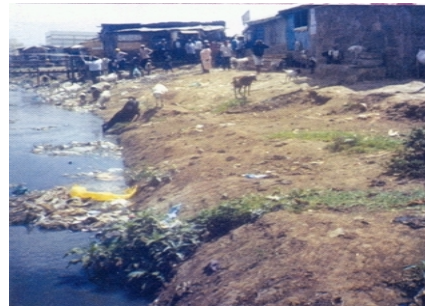
Figure 8: Mukuru - Sewer lines not present and solid waste dumping in Ngong River
