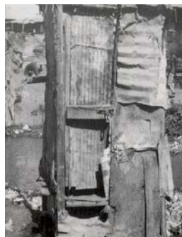
Figure 10: Informal community toilets
