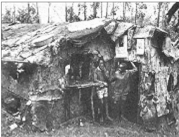
Fig. 5. An informal structure pole/timber frames covered with paper/plastic/cardboard recycled sheets (Hake, 1977).
