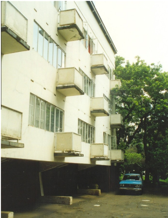
Fig. 12. External view of Delamere Estate block (Makachia, 2010).
