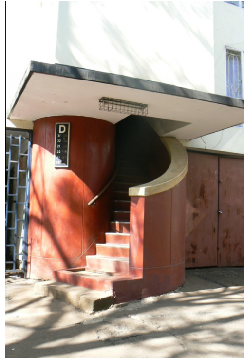
Fig. 13. Staircase detail in Delamere Estate (Makachia, 2010).
