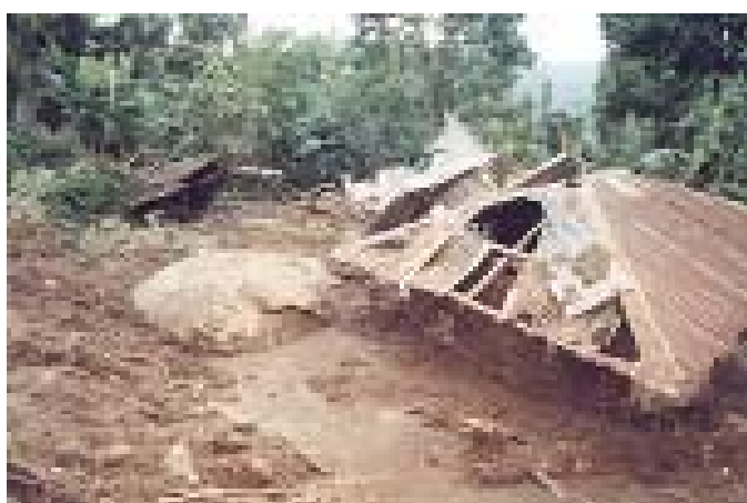
Plate 2: Flood damage in Western Kenya
