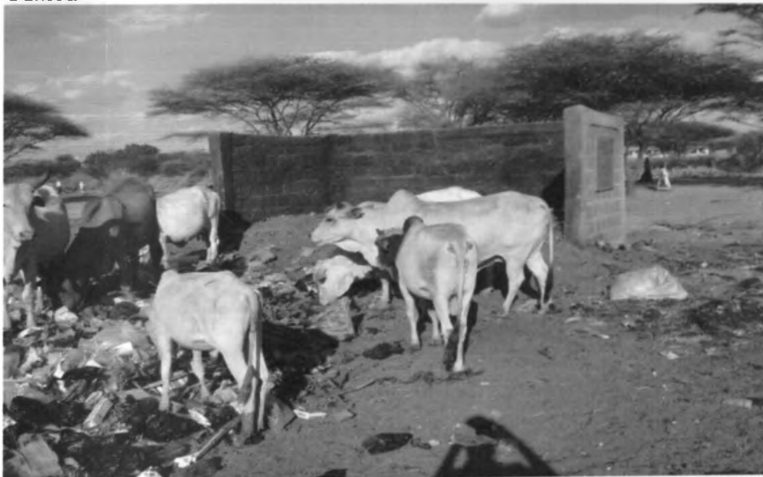
Plate 5-5 : An overwhelmed Refuse Chamber next to Catholic Church, Garissa
