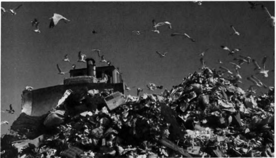
Plate 2 – 7 ; A Landfill Operation in progress
