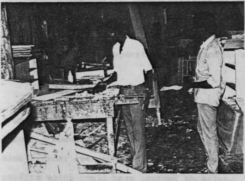
b. Carpenters at work; work spaces are generally congested.
