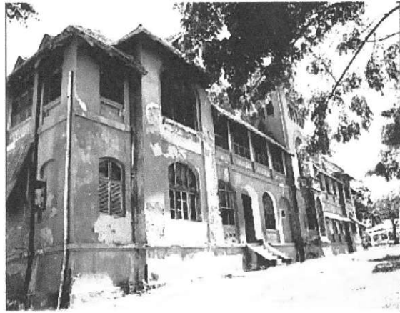
Plate 4.13: Peeling off of wall due to climatic condition [cliff block/
