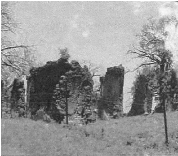
Plate 4.5: Tongoni ruins very fragile, some of the walls have a lot of cracks and peeling off of plaster.
