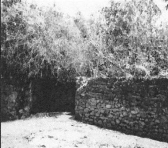
Plate 4. 2: Kwale defensive wall without Plaster
