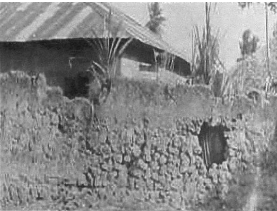
Plate 4.4: Deterioration due to climatic condition. Part of Chongolian defensive wall
