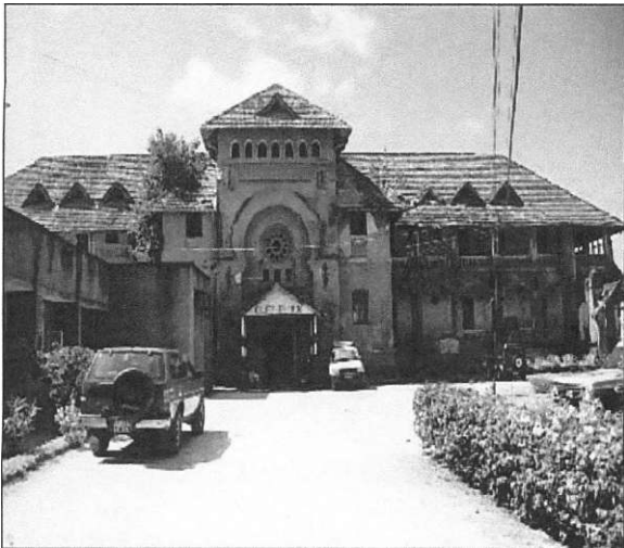
Plate 4.12: Front view of Cliff block,, deterioration caused by climatic condition (Growth of plant ) On the left there was extension of new building.
