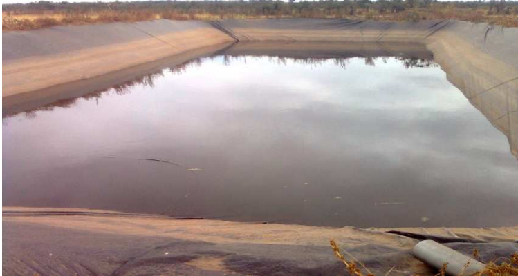
Plate 4.1 A water pan lined with polythene sheet to reduce seepage loss
