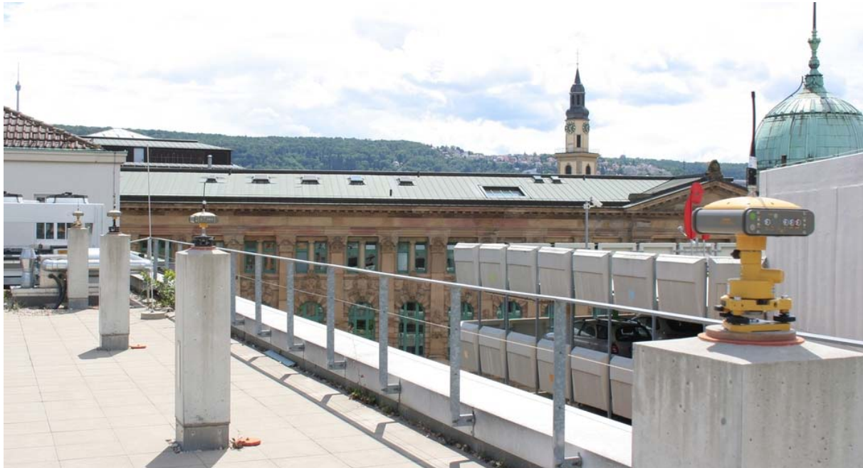
Figure 2: Pillars on the roof of HFT Stuttgart building 2 equipped with dual frequency GNSS receivers TOPCON Hiper Pro.
