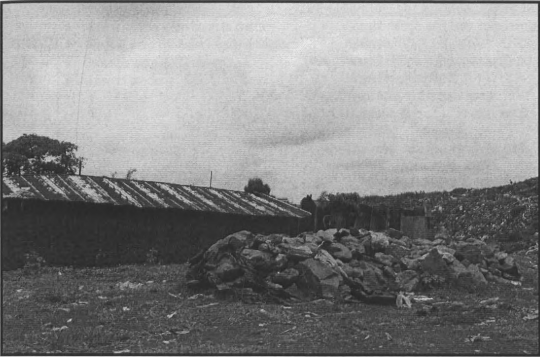
Photo: This house has in Grogan B has been constructed in a flood plain for Nairobi River. An artificial dyke is used to break the flood waters during the rainy seasons. (Source: Fieldwork)
