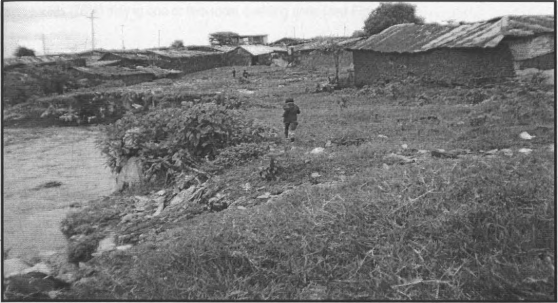
Photo : School located close to the river bank, exposing pupils to vulnerabilities related to flooding during the rainy seasons (Source: Fieldwork)
