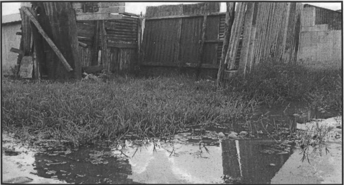
Photo: This area has been rendered uninhabitable due to constant inundations with flood water. Notice the neglected house structures. (Source: Fieldwork)
