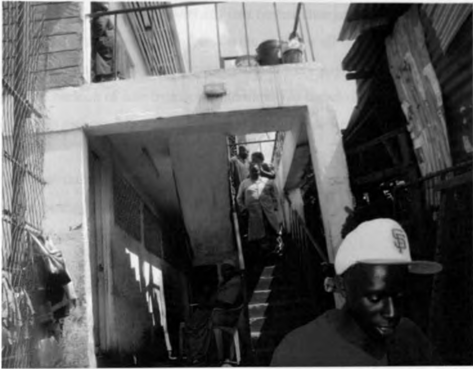
Figure 10: Kamukunji Jua Kali Association office (upstairs) and ablution (downstairs) block. The block also has a boardroom/hall where various associations affiliated to the KJKWA meet.
